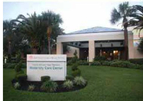
TOP: The Miriam and Hugh Nunnally Health and Science Building; ABOVE: The Miriam and Hugh Nunnally Center for Maternity Care
